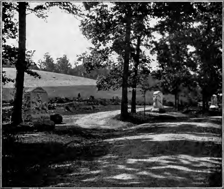
Near Widow Glenn House, Looking North Toward Bloody Pond
